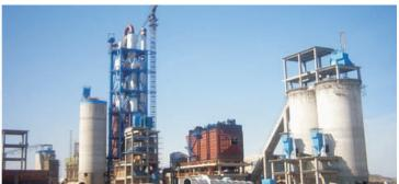
The whole production process of cement is generally as follows: homogenizing-- preparation of raw material -- raw material homogenization -- preheat decomposition -- the burning of cement clinker -- cement grinding mill -- cement packaging. In the process flow, different cement making machines should be used.
