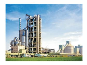
Cement grinding station is composed of dust collector, bucket elevator, belt conveyor, spiral conveyor, high efficiency ore dressing machine and so on.
